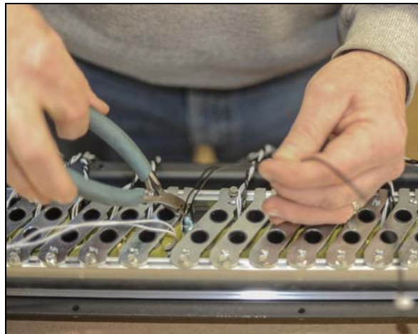
Illustration 121 - Cutting wires on unused solenoids.
