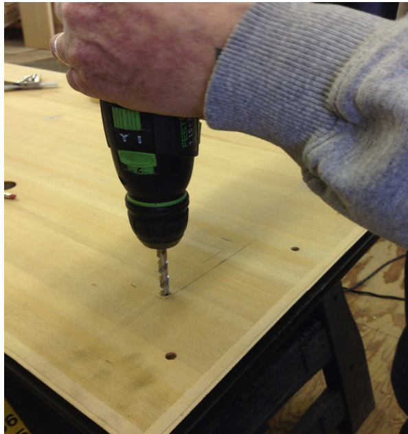
Illustration 49 - Drilling corners
